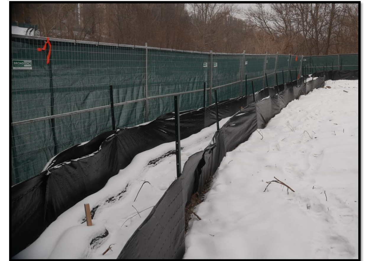
Double silt fencing at the elevated guideway construction site
