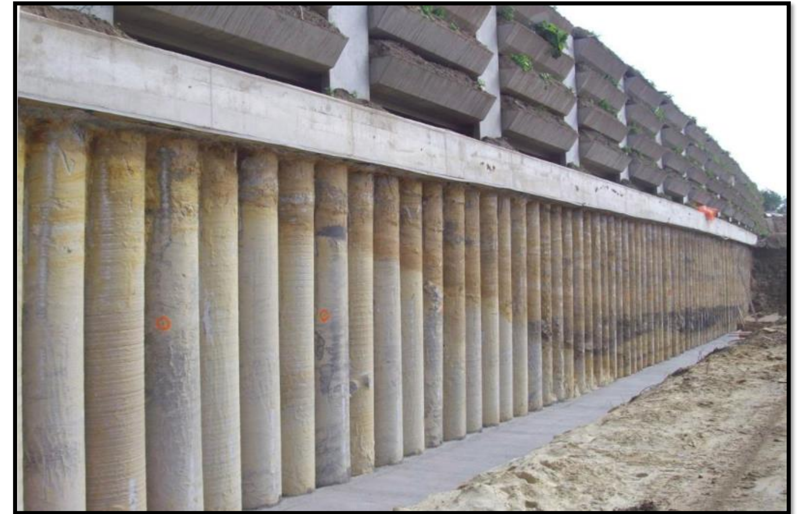
Example of secant pile wall Source: www.geotech.hr
