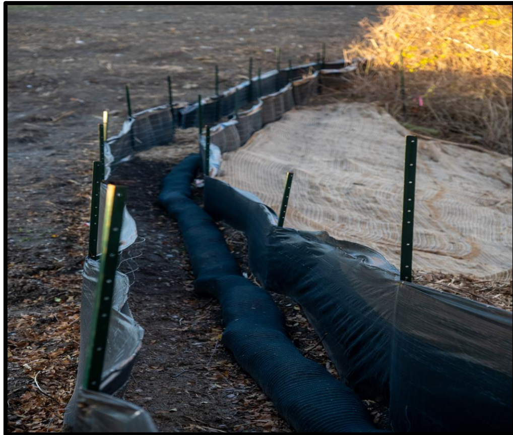
Coir log installed at the elevated guideway construction site
